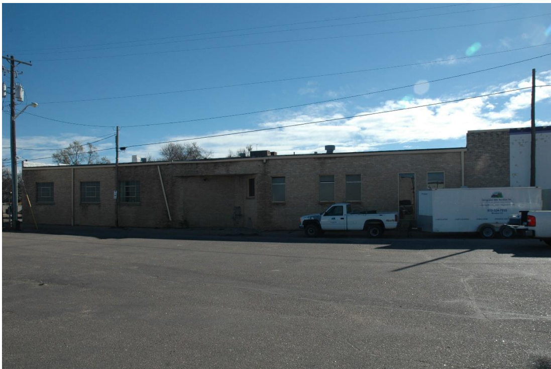
CD 2, Image 9, View to SSE of rear portion of north side
