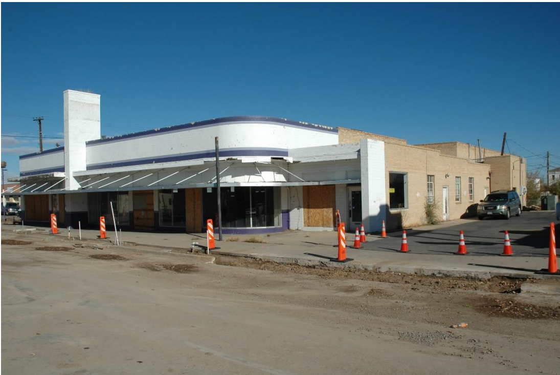
CD 2, Image 5, View to NE of façade (west) and south side
