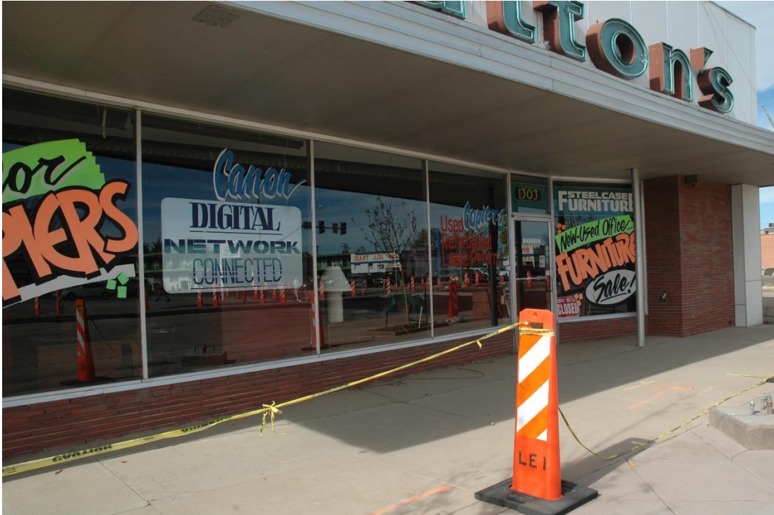
CD 1, Image 64, View to NW of lower façade (east)
