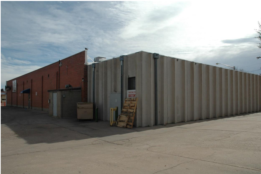
CD 1, Image 65, View to SE of north side and north and west sides of the addition
